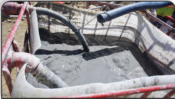
1 Return drilling fluid transferred to desilter cone manifold for cleaning
