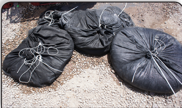
6 Bagged solids removed and set aside for proper disposal
